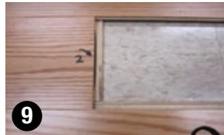
**9-** At the end of the board remaining in the floor, apply a small bead of glue to the groove in the tongue just in front of the plastic receptor. (See side #2)
