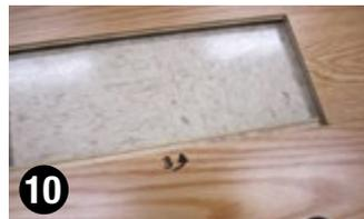
**10-** Apply a small bead of glue to the groove in the tongue along the length of the board remaining in the floor. (See side #3)
