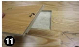
**11-** Apply a small bead of glue along both the end of the board in the floor and the newly cut piece. (See side # 4)
