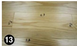
**13-** Once the new board is installed, place sufficient weight on top of the board to maintain it in place for 24 hours while the glue dries.
